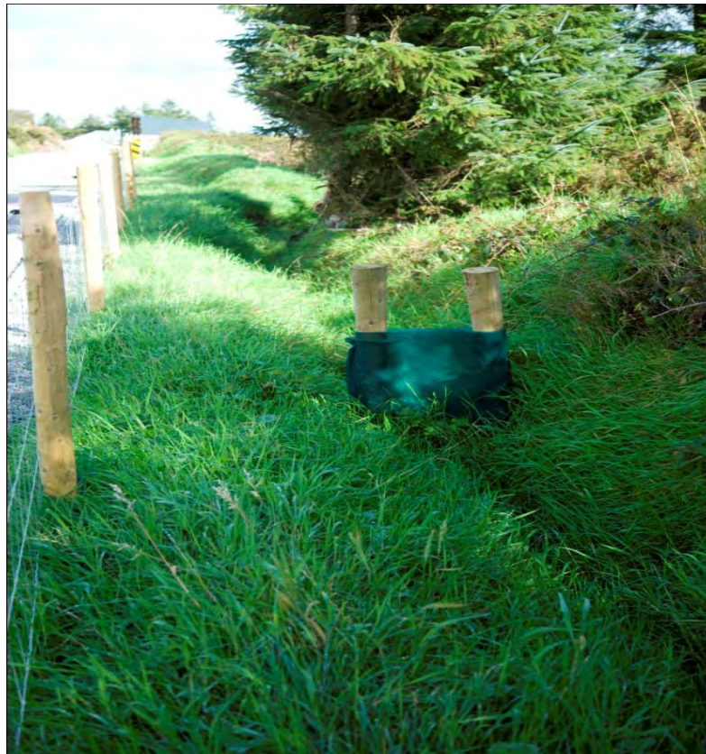
Figure 4.4: Typical Silt Trap across Grassed Swale
